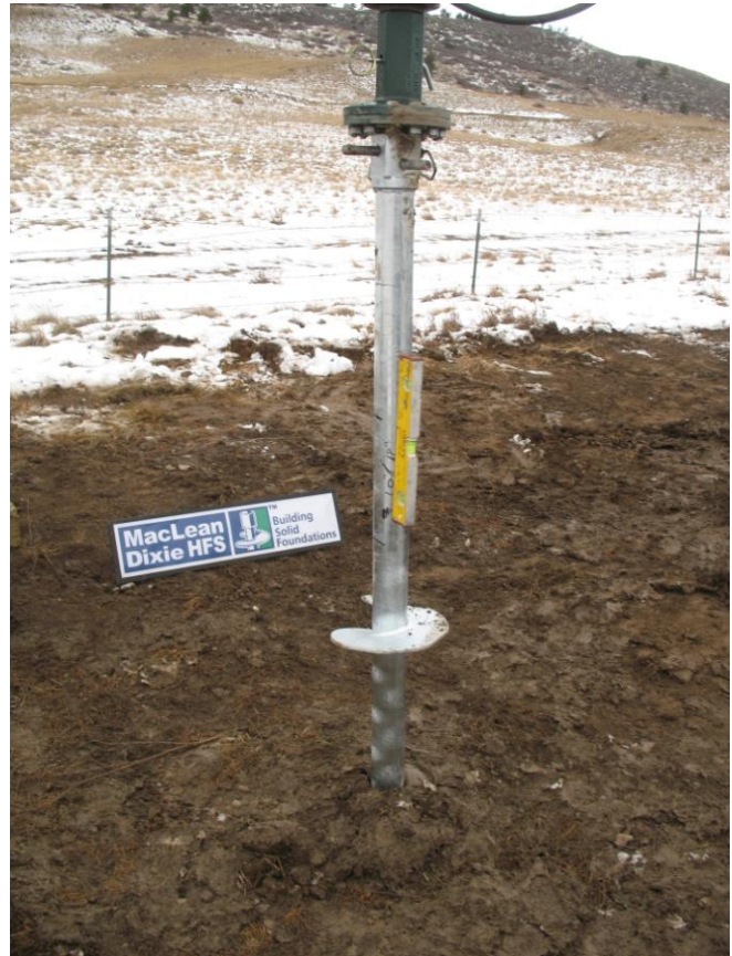
Installing Pipe Shaft Foundation Pile/Anchor
