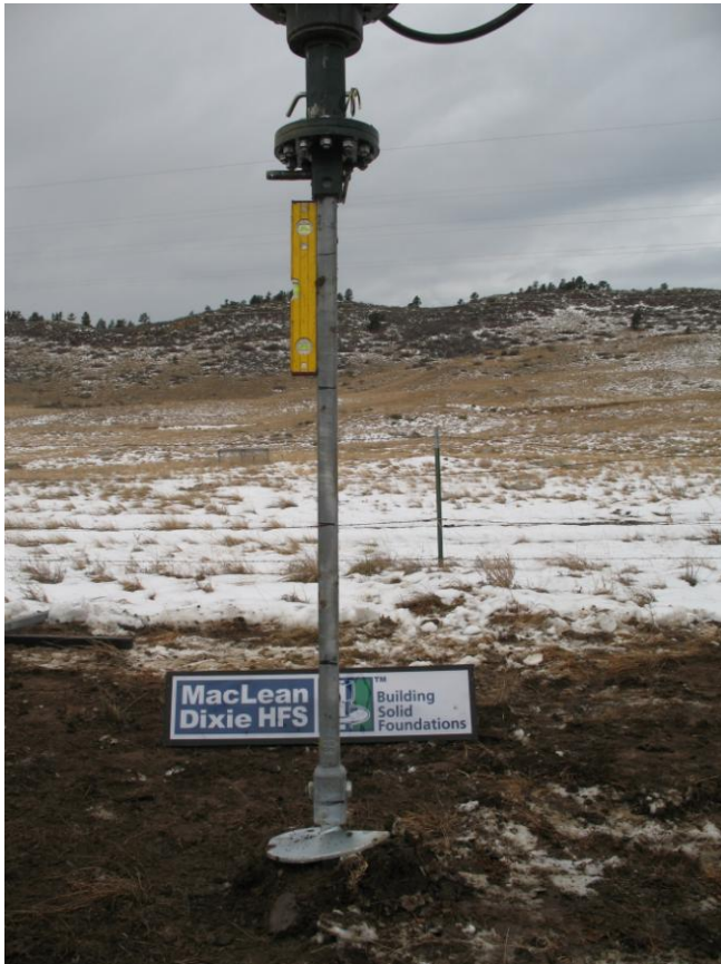
Installing RCS (Round Corner Square) Shaft Foundation Pile/Anchor
