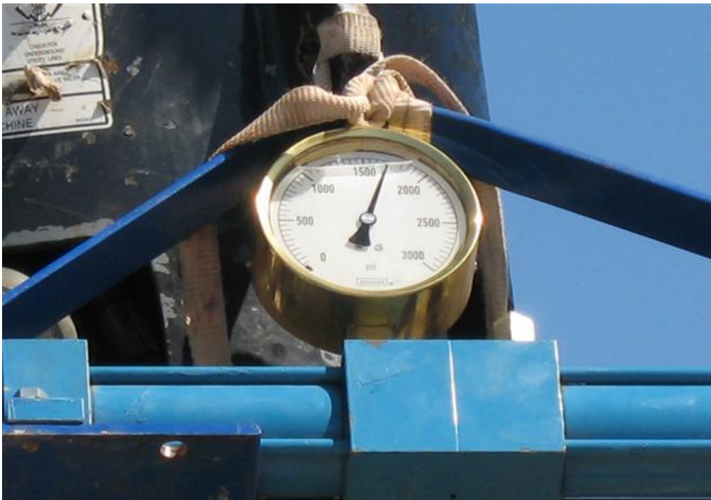
Typical calibrated hydraulic gauge (PSI) and converted to torque used to measuring installing torque.
