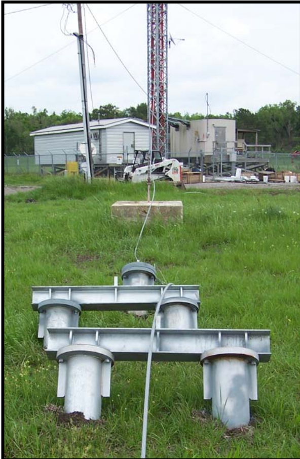
Single and tandem installed CHPP piles for the guys. The cross beam was bolted to the tandem anchors
